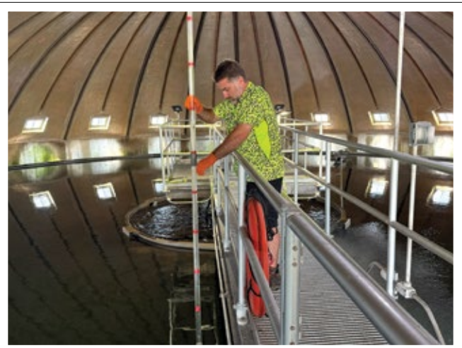
Brandon Scurto Clarifier Blanket Level
