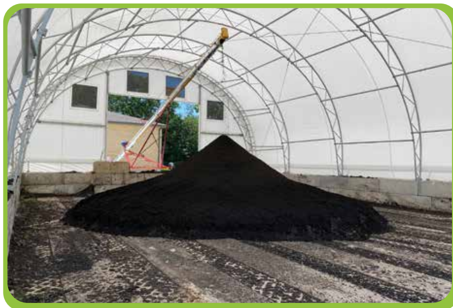
Sludge Conveyor and Stockpile
