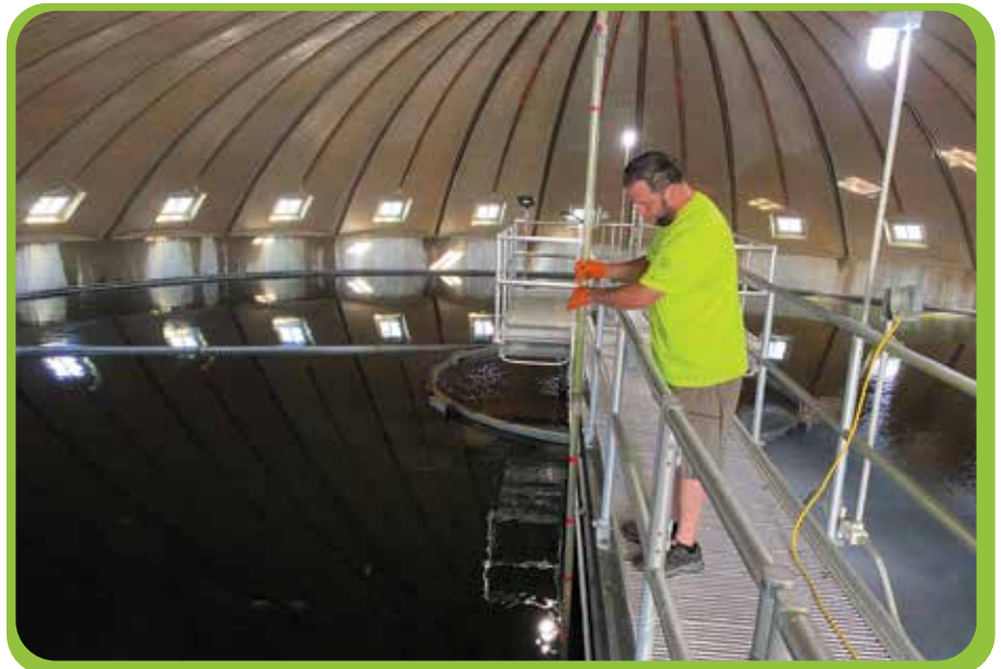
Operator Chris Molidor Measuring Sludge Blanket
