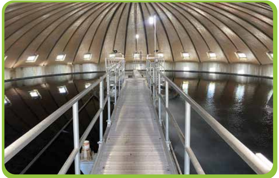
Rebuilt North Clarifier
