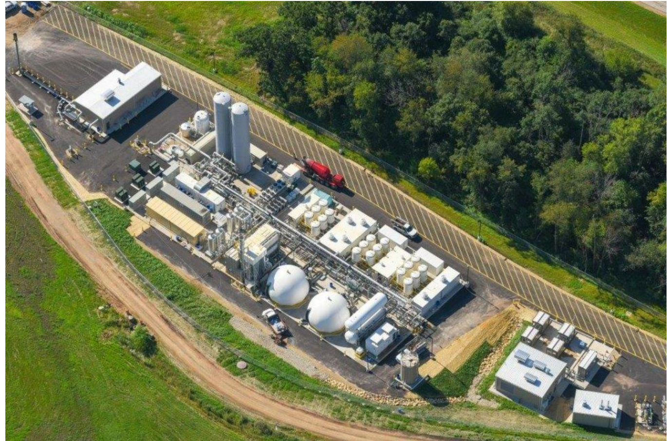
Dane County Rodefild Landfill RNG Facility
